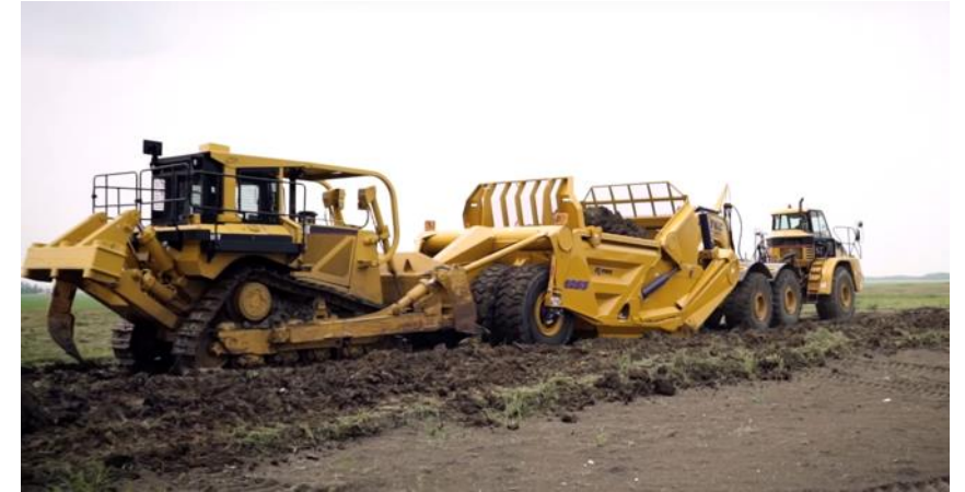
Removing topsoil with scraper
