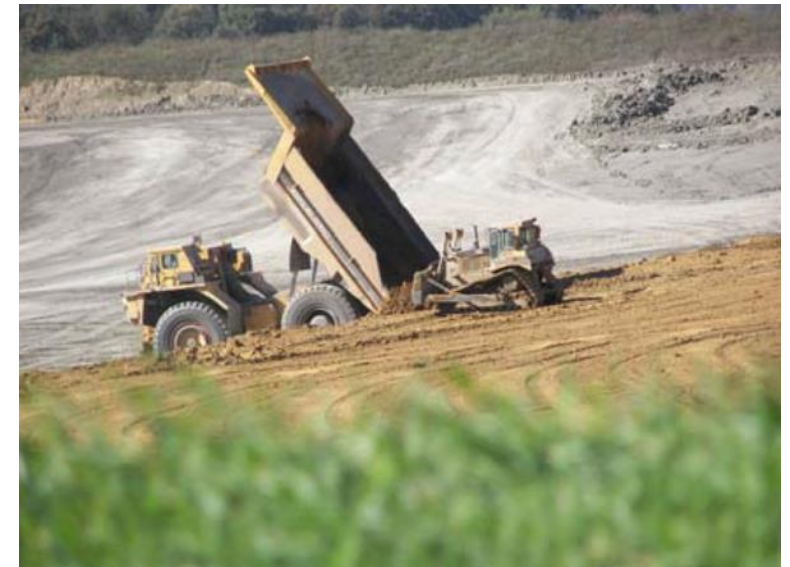
Backfilling and grading subsoil
